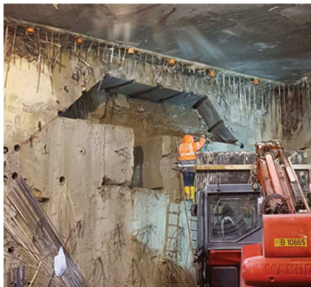
Figure 12. Diaphragm wall during cutting.
