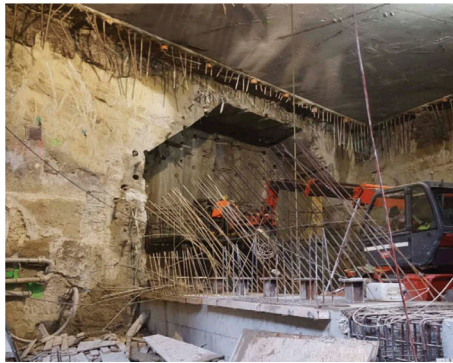
Figure 11. Diaphragm wall after cutting.
