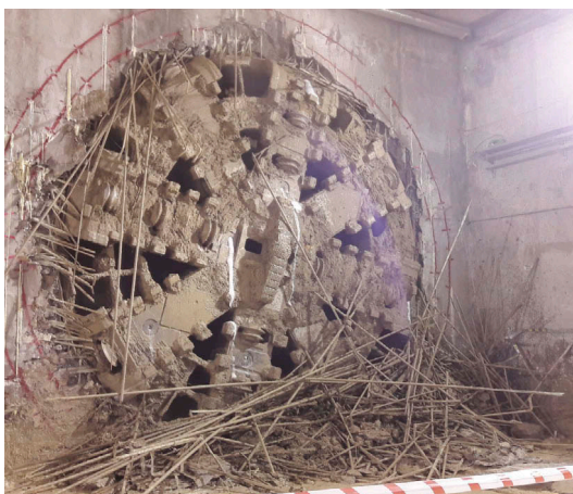
Figure 5. Break-through of the Left TBM at C15 station.
