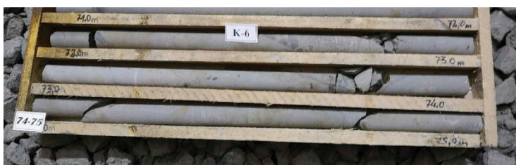
Figure 4. Magura strata – good core of rock in main tunnel.
