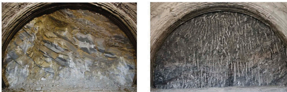
Figure 7. Front face with sandstone and shale (on the left), shale (on the right).
